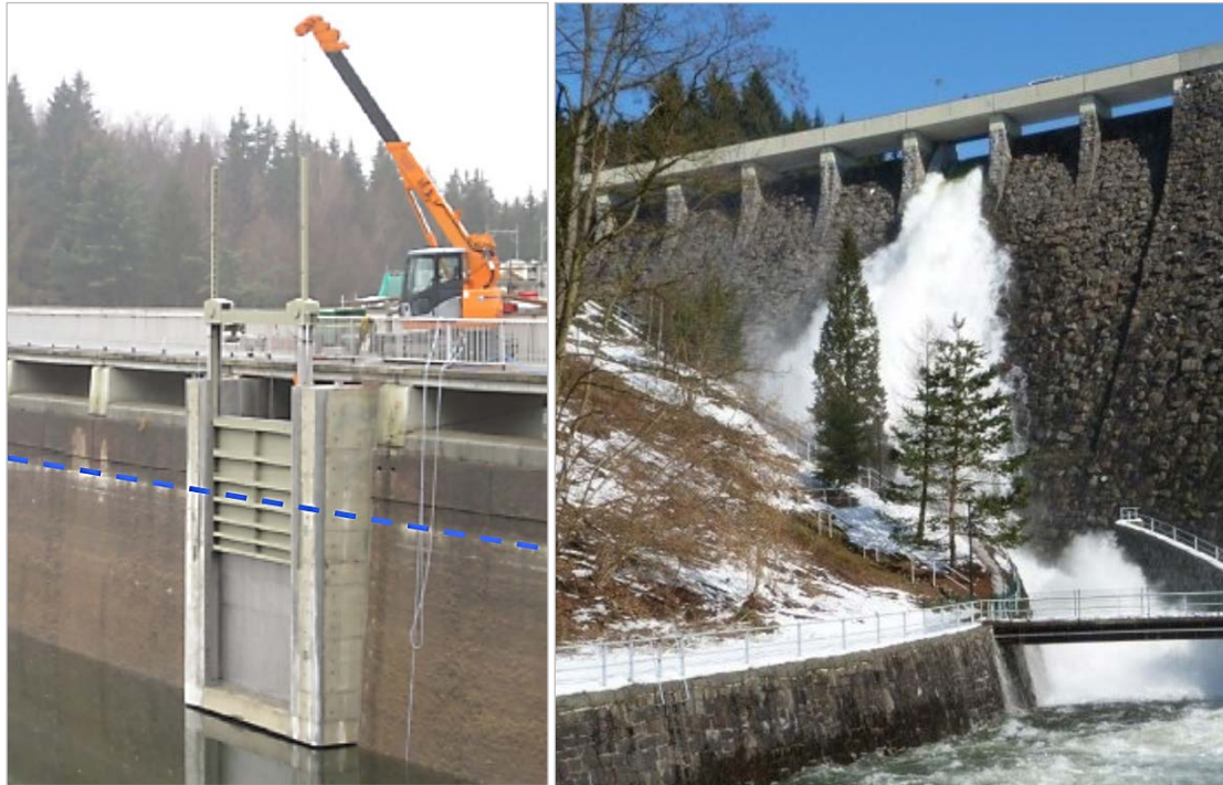
Figure 2: Surface outlet structure. Left: Vertically movable penstock allowing to adjust overflow level (blue line: flood control fill level); right: functional test at approximate maximum outflow capacity of the outlet (10 m 3 /s). Photos: LTV
